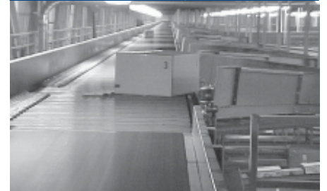
Photograph 3. High speed sortation conveyor
