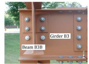
View C. Double bolted-welded-angle shear connection, back of View B
