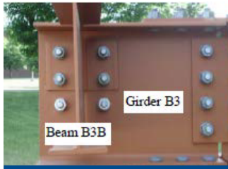
FIGURE 1c. Double bolted-angle shear connection, back of view 2
