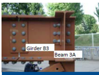
FIGURE 1b. Double bolted-angle shear connection, view 2
